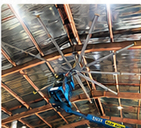
Exxonmobil Warehouse Kemaman
